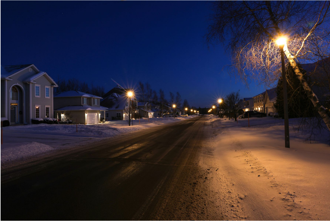
Before: 100W High Pressure Sodium HID Lamps
